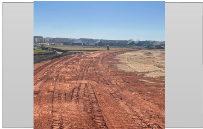
Baseball field warning track being installed
