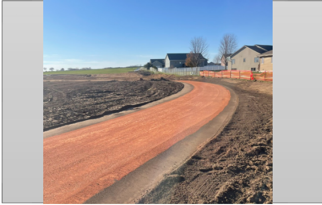
Softball field warning track installed
