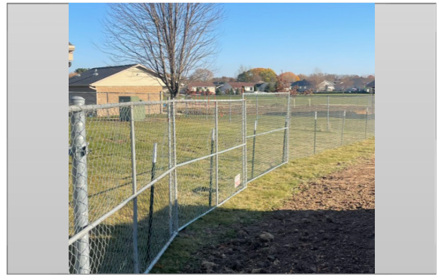
Temp fence installed on backside of pump house
