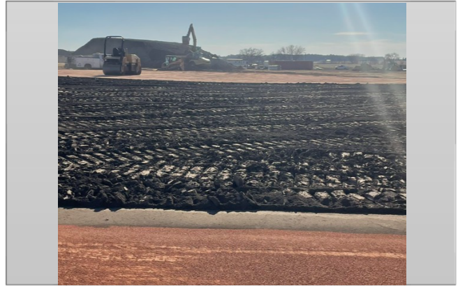
Softball outfield shredded topsoil and infield sand being installed
