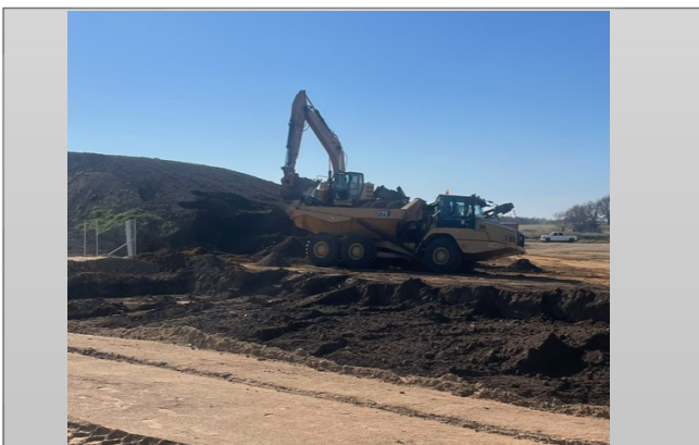
Topsoil being shredded and loaded into a truck
